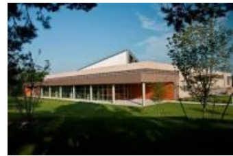
Emerson’s new state-of-the-art and energy-efficient global data center in St Louis
